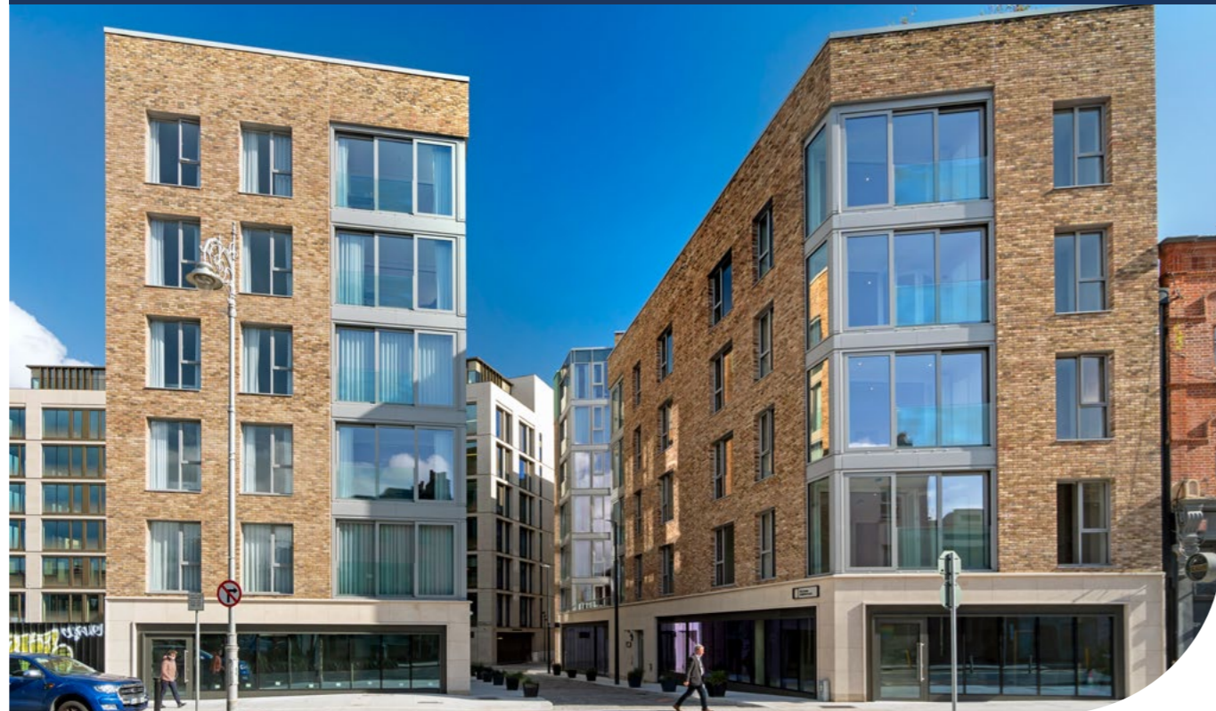
Charlemont Square Blocks 5 & 7: Dublin
